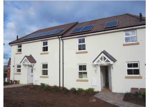
Picture 12 Photo-voltaic roof panels
